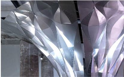
Fig. 2. The “Arum” surface was designed by Zaha Hadid Architects in cooperation with Robofold for the 2012 Venice Biennale. It consists of metal sheets folded along curved creases.
