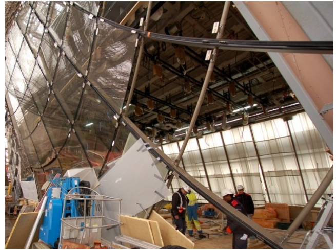
FIGURE 3.13: The Eiffel Tower Pavilions feature beams with rectangular cross-section whose side flanks are manufactured by bending. This makes them developable, and makes the entire beam arrangement a semidiscrete version of a principal support structure (image: Evolute).
