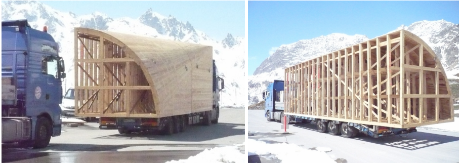
FIGURE 4.4: Formworks for concrete. The wooden structure fills a quarter of a tunnel (the remaining three quarters are filled by similar constructions). It connects a circular opening with a rectangular one. The outer surface of the formworks is a developable defined by boundary curves C_1 , C_2 where C_1 is a circle and C_2 is a rectangle. In this special case the developable is part of \partial \text{co}(C_1 \cup C_2) (Silvretta reservoir, Austria. www.spezienschalungen.com ).
