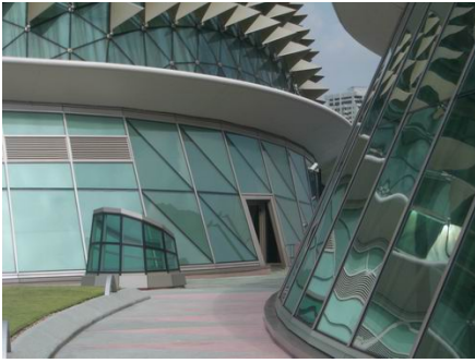
FIGURE 3.10: Doubtless these non-planar quads were subdivided after the design phase.
