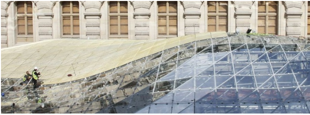
FIGURE 3.11: Polyhedral surface in the Louvre, Paris, by Mario Bellini Architects and Rudy Ricciotti, during construction. It has only as many triangular faces as are necessary to realize the architect's intentions, and as many quadrilateral faces as possible in order to lighten the load and reduce the number of parts.
