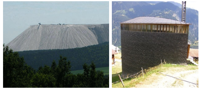
FIGURE 1.16: Spoil tip of the Heringen potash mine (Germany), and the chapel of S. Benedetg (Sumvigt, upper Rhine, Switzerland). These constant-slope surfaces, hence developable.
