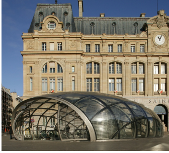
Figure 22: Repetition aides manufacturing efficiency. The lentille at Saint Lazare metro station is composed of a sphere and a torus, and has a rotational symmetry no longer apparent after panelization. This symmetry enabled the reuse of molds used in the manufacturing of glass panels (engineering and photo: RFR).
